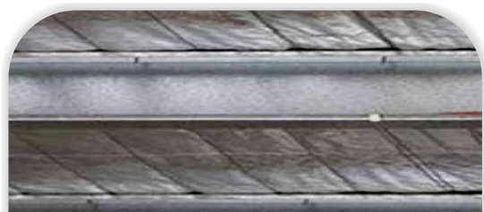
ROOFING AND WALL/CLADDING
